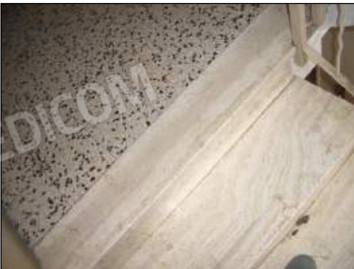
Vista scale condominiali
